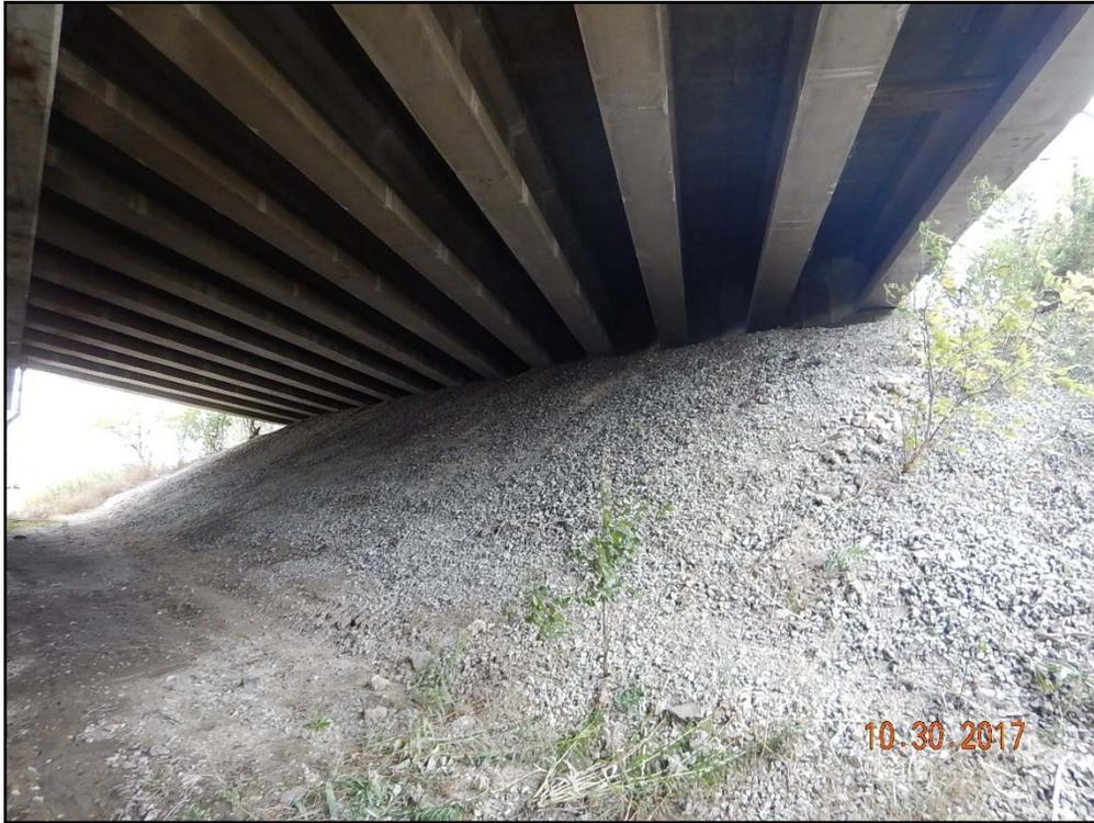
Photo 37: Waukegan Road, typical crushed stone slope wall, north slopewall shown
