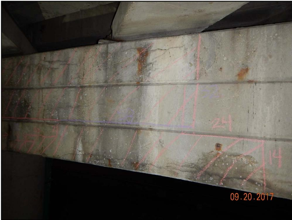
Photo 27: Waukegan Road, full height delamination, pier 2 cap
