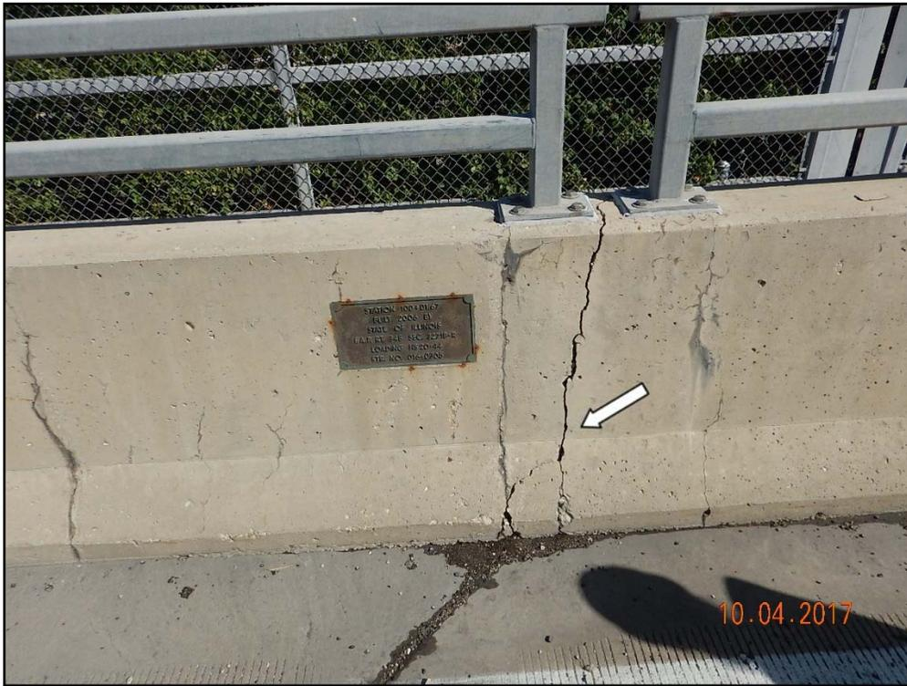
Photo 13: Waukegan Road, crack in the parapet due to no expansion joint at the south abutment
