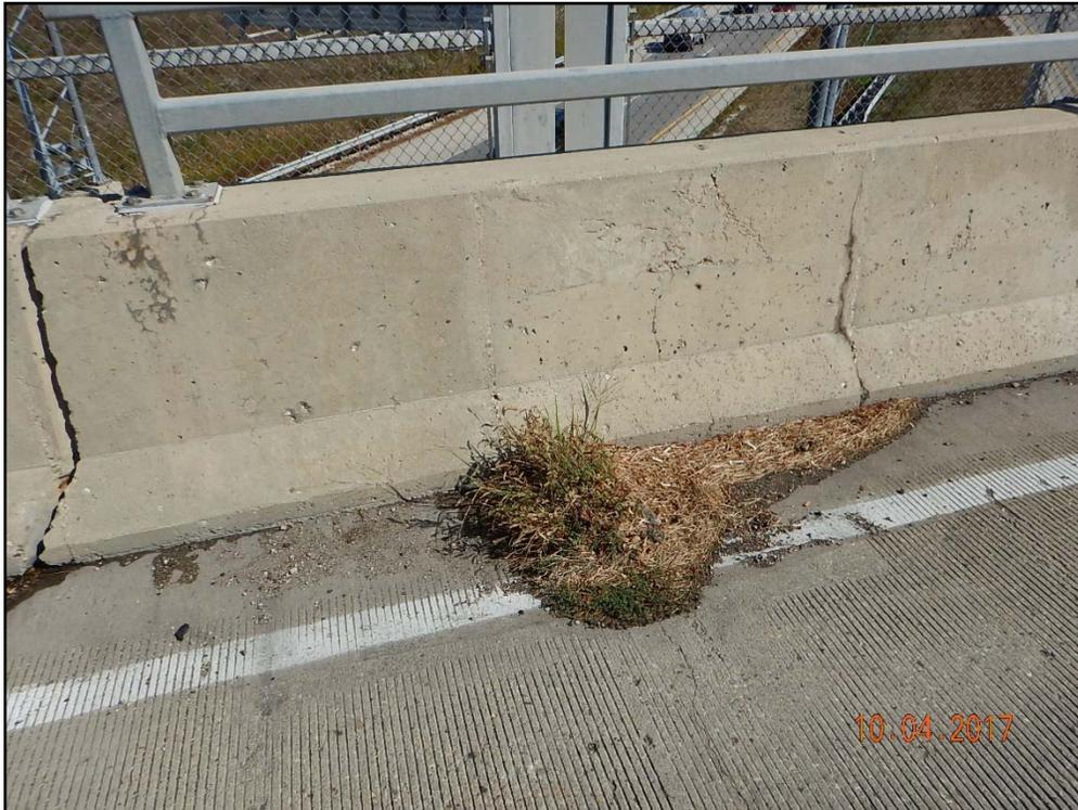
Photo 34: Waukegan Road, typical clogged scupper drain
