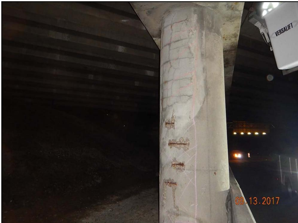
Photo 22: Waukegan Road, delaminated previous repair with map cracking and water penetration, column 5 of pier 1 shown
