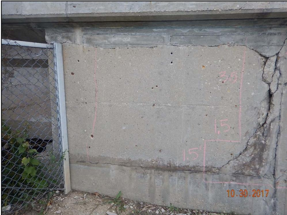
Photo 38: Waukegan Road, typical wingwall spall, northeast wingwall shown
