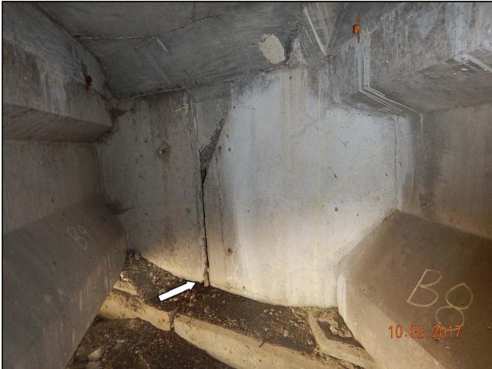
Photo 36: Waukegan Road, PJF protrudes roughly 3" out of the joint, south abutment
