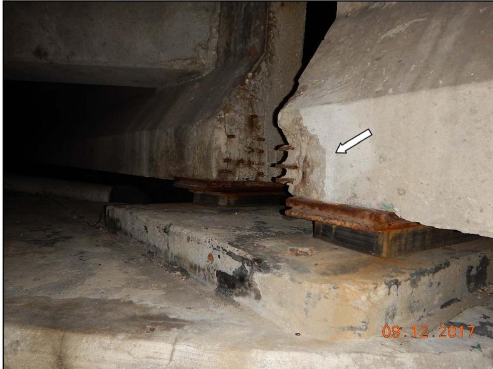
Photo 14: Waukegan Road, typical spalled beam ends at the piers, beam 1 at pier 1 shown
