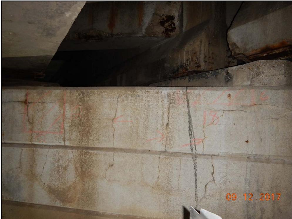
Photo 24: Waukegan Road, vertical cracking on the pier cap between beam 5 and 7, pier 1
