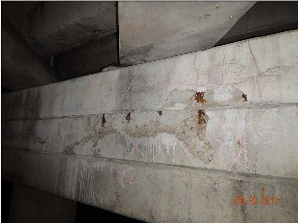
Photo 28: Waukegan Road, spall with exposed reinforcement, pier 2 cap
