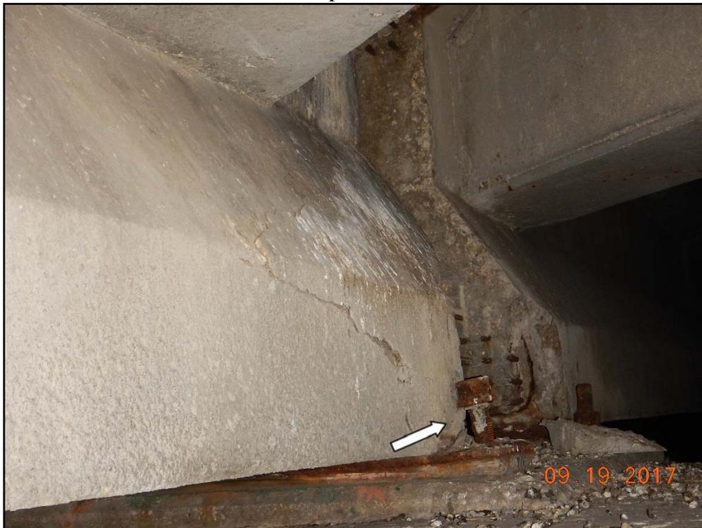
Photo 20: Waukegan Road, loose bearing plate anchor bolt for beam 2 at pier 2
