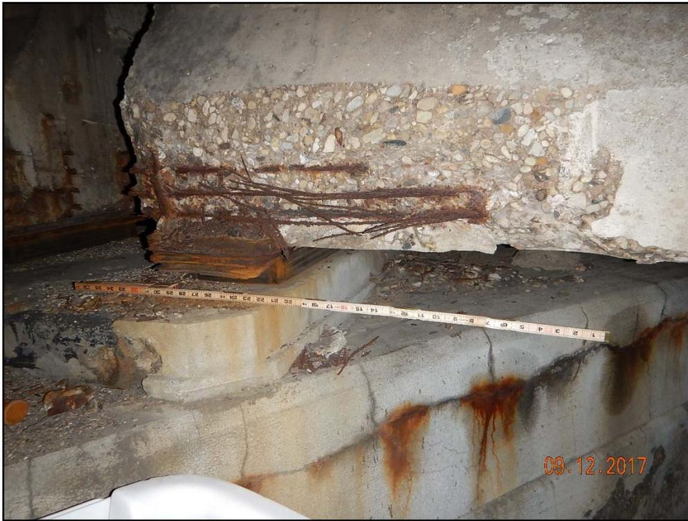
Photo 17: Waukegan Road, spall with exposed and frayed prestressing strands, bottom flange of beam 5
