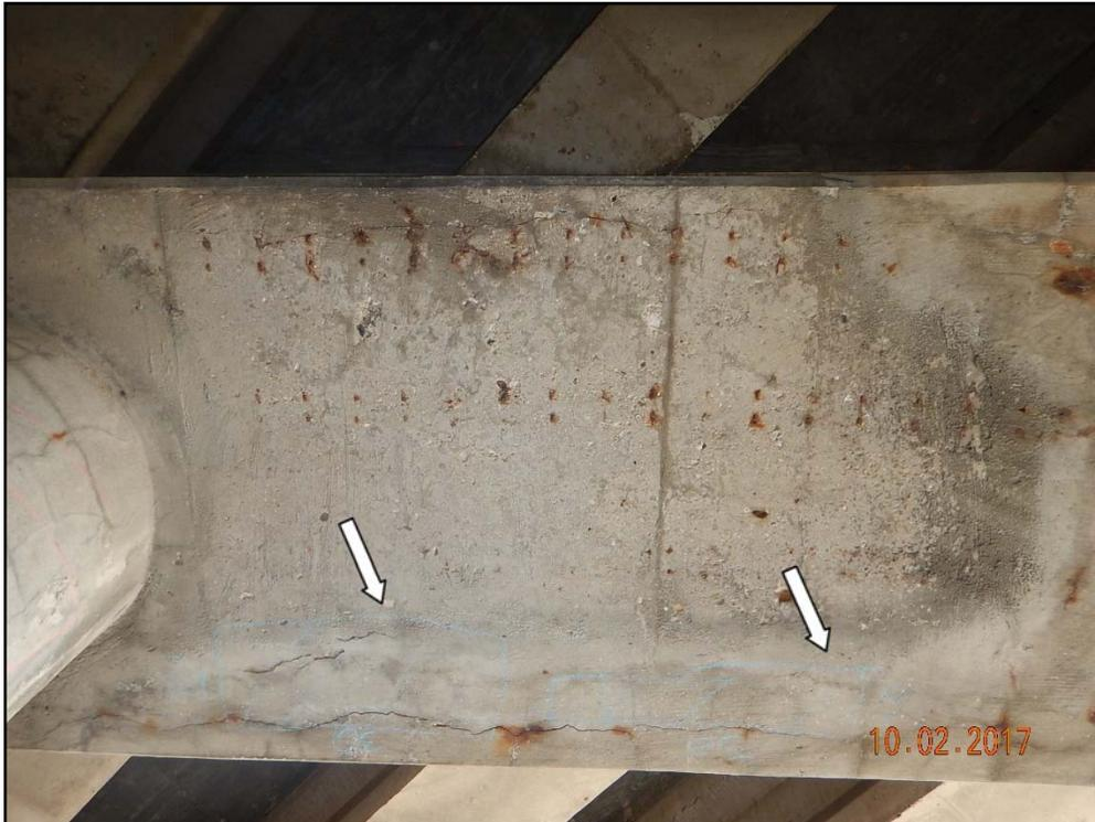
Photo 26: Waukegan Road, delamination, underside of pier 1 cap
