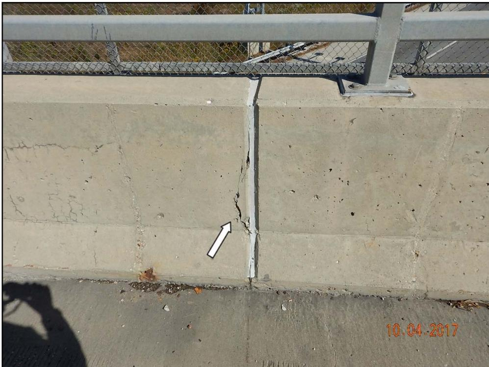
Photo 12: Waukegan Road, typical cracking in the parapet at expansion joints
