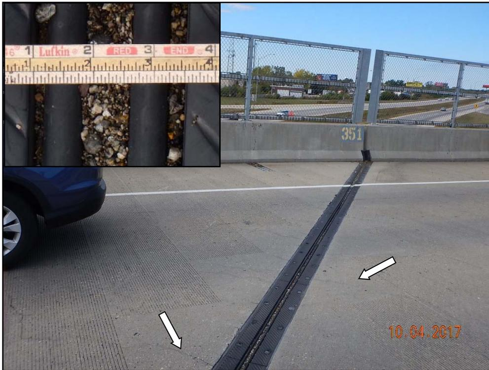
Photo 2: Waukegan Road, pier 1 expansion joint with diagonal cracking (Looking West)
