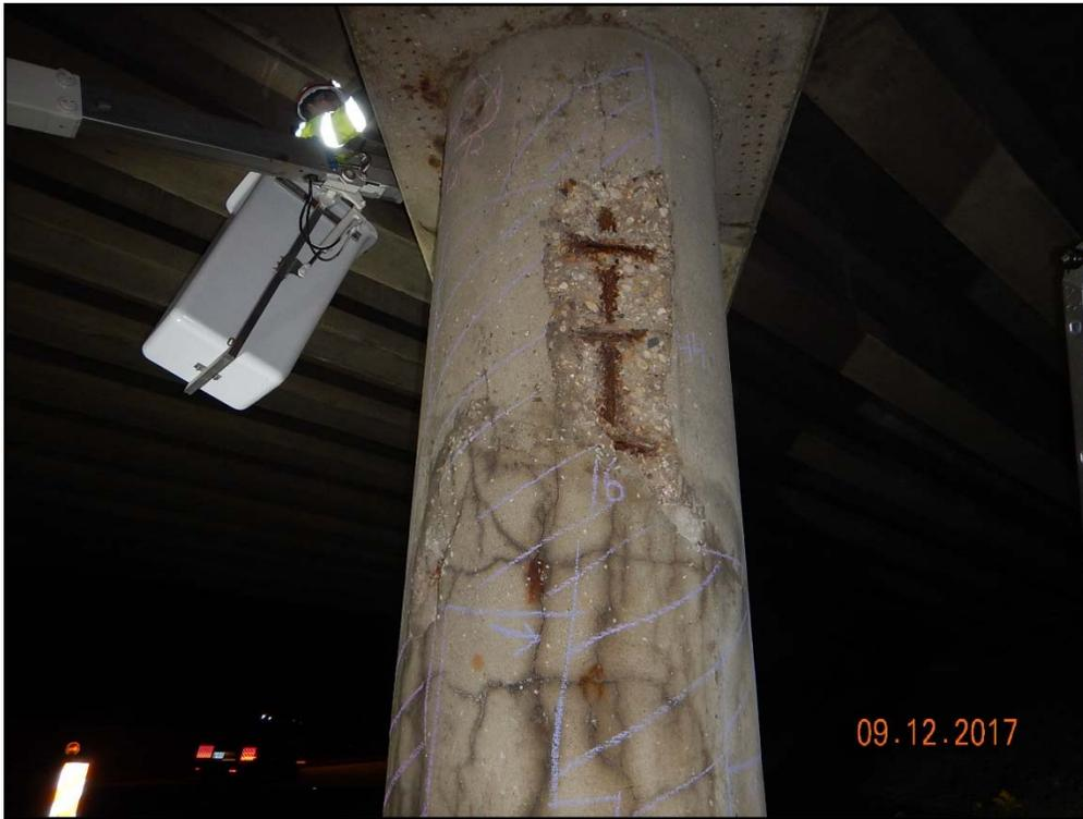
Photo 23: Waukegan Road, spall with exposed reinforcement, column 2 of pier 1 shown
