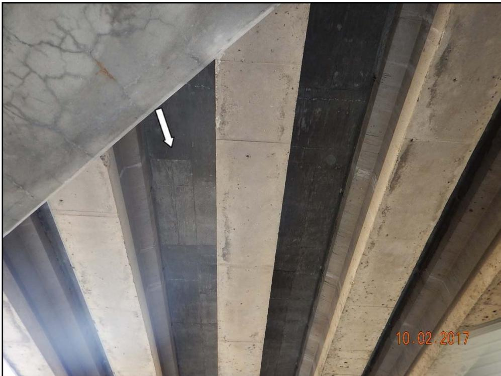
Photo 10: Waukegan Road, full depth deck repair, span 2
