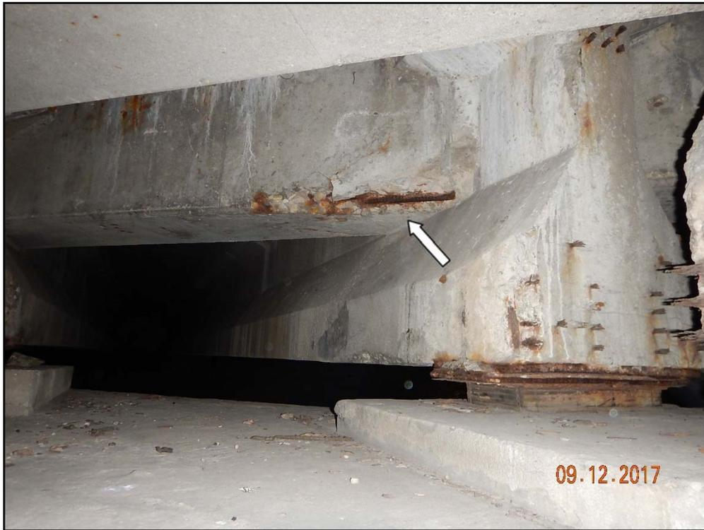
Photo 15: Waukegan Road, typical spalled diaphragm
