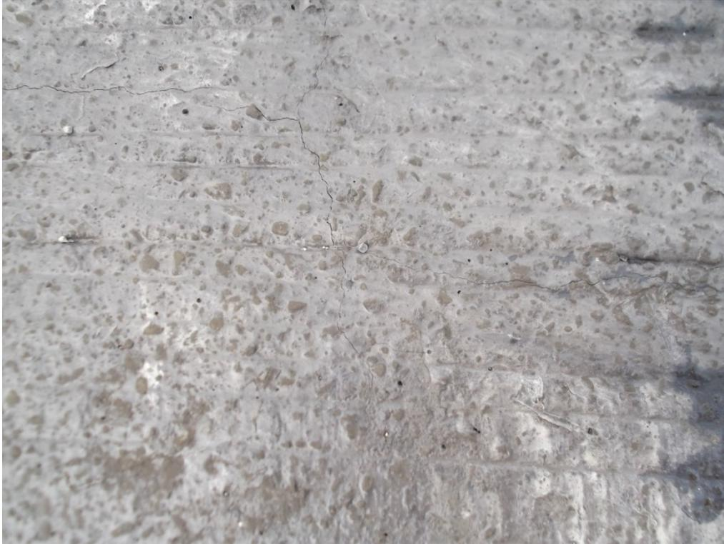
Fig. 7 – Cracks meeting at center of patch.
