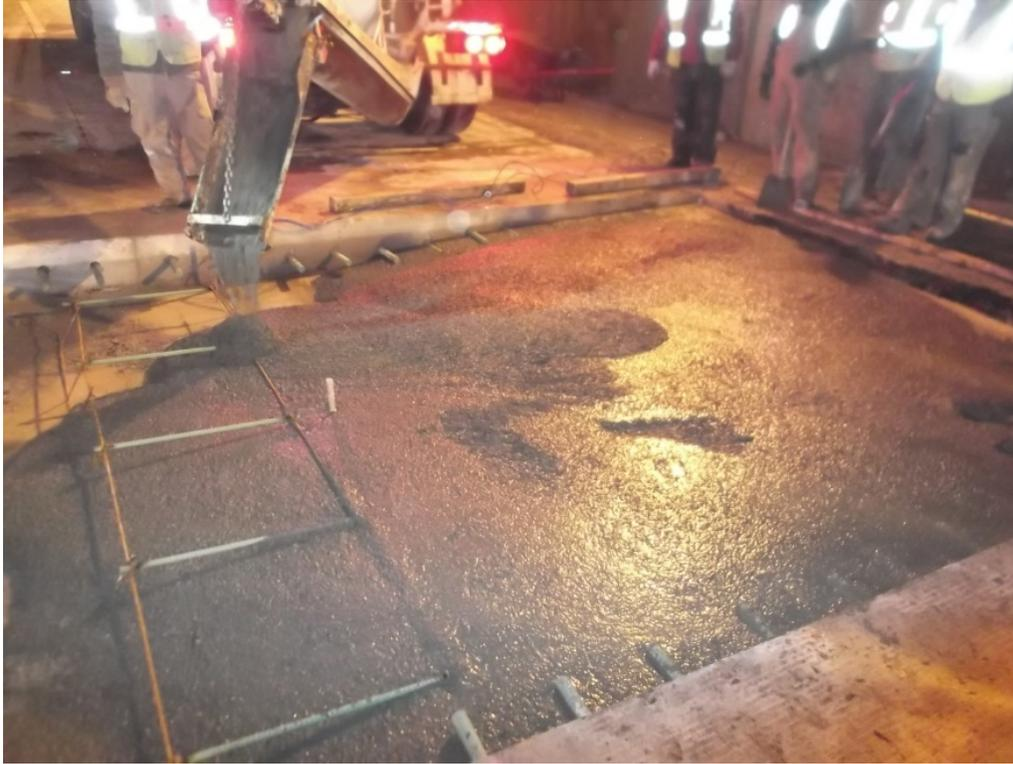
Fig. 29 – Concrete placement at patch 3.
