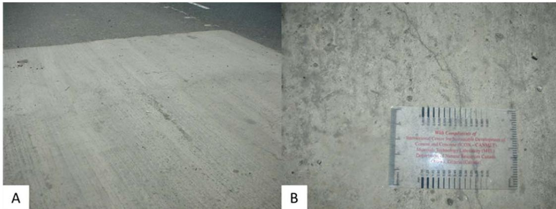
**Figure 2-5 – Full-Depth CAC Repair on I-290, Chicago, IL: (A) Overview, (B) Cracking**
