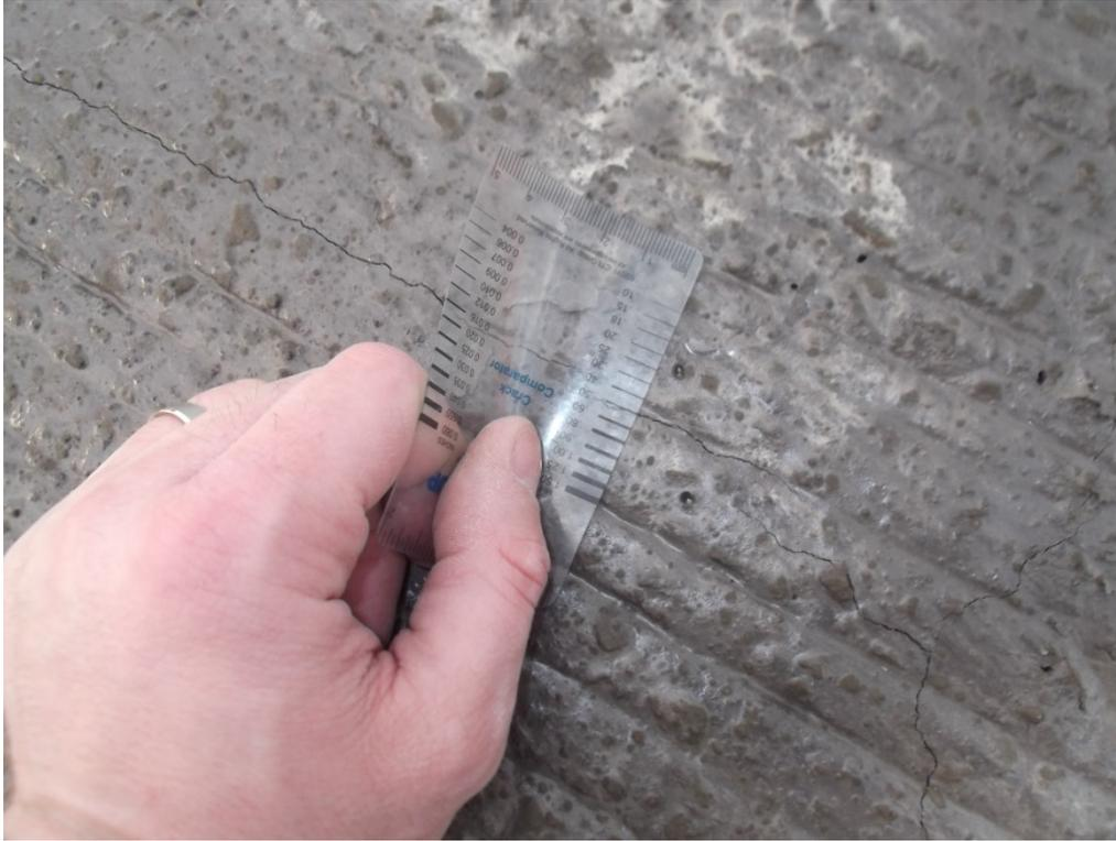
Fig. 9 – Transverse crack (0.50mm).
