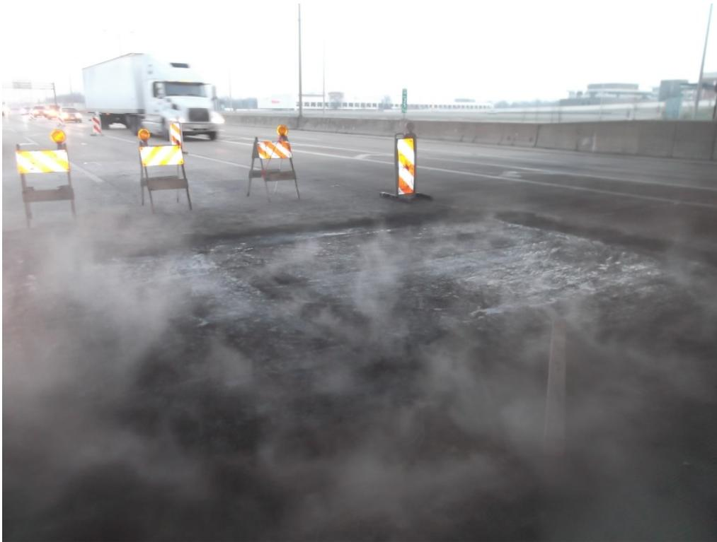
Fig. 32 – Finished patch 3 (after removal of plastic, before saw-cutting).
