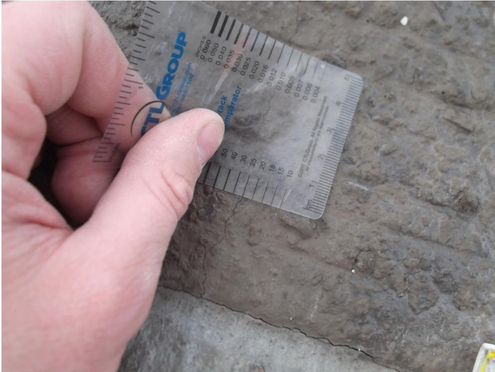
Fig. 8 – Longitudinal crack at south edge (0.25mm).
