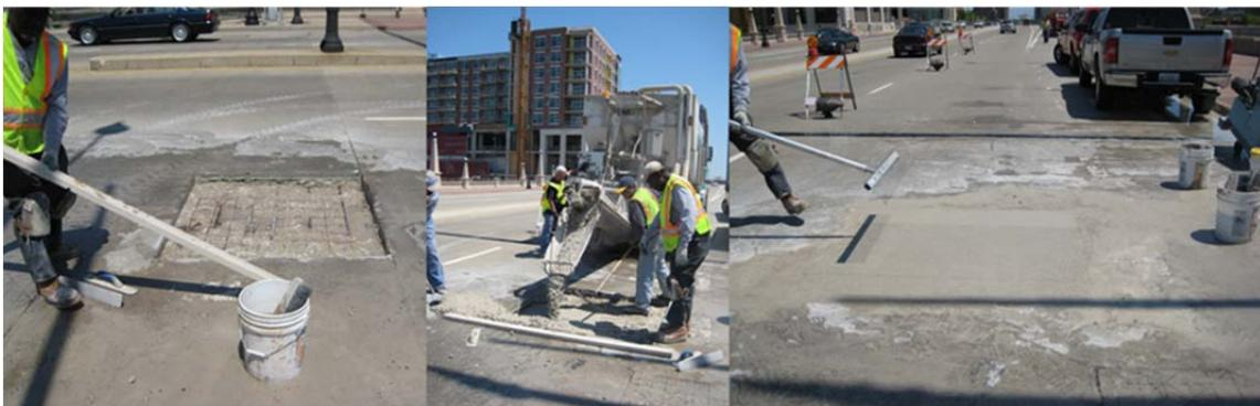
**Figure 2-6 – Partial-Depth CAC Repair, Roosevelt Bridge, Chicago, IL**
