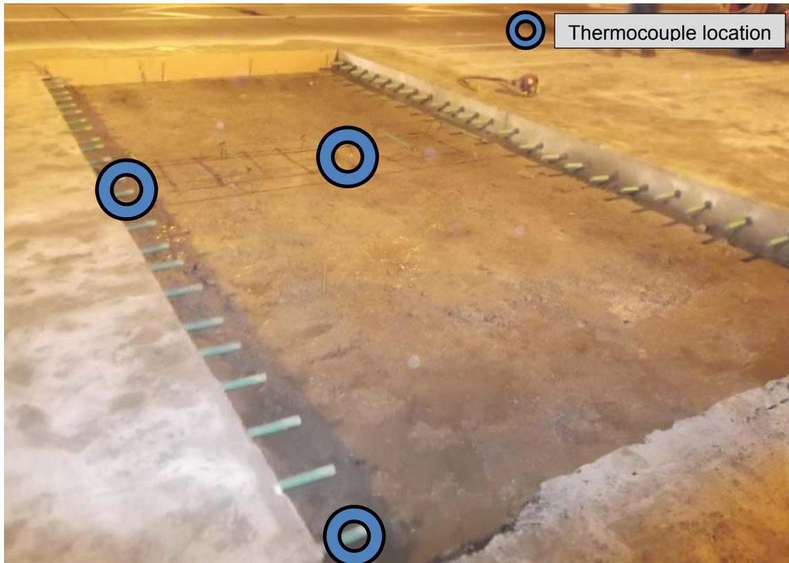
**Figure 3-30 – I-294 Patch, Repair Area**
