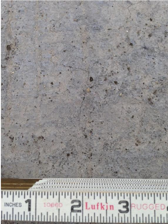
Fig. 18 – Cracking observed in non-accelerated portion of patch 2.
