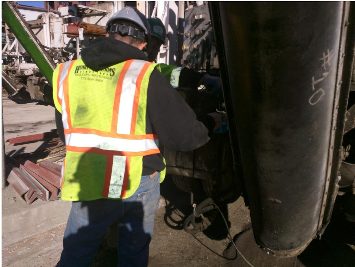
Figure 3 - Dispensing Accelerator for Calibration Procedure.
