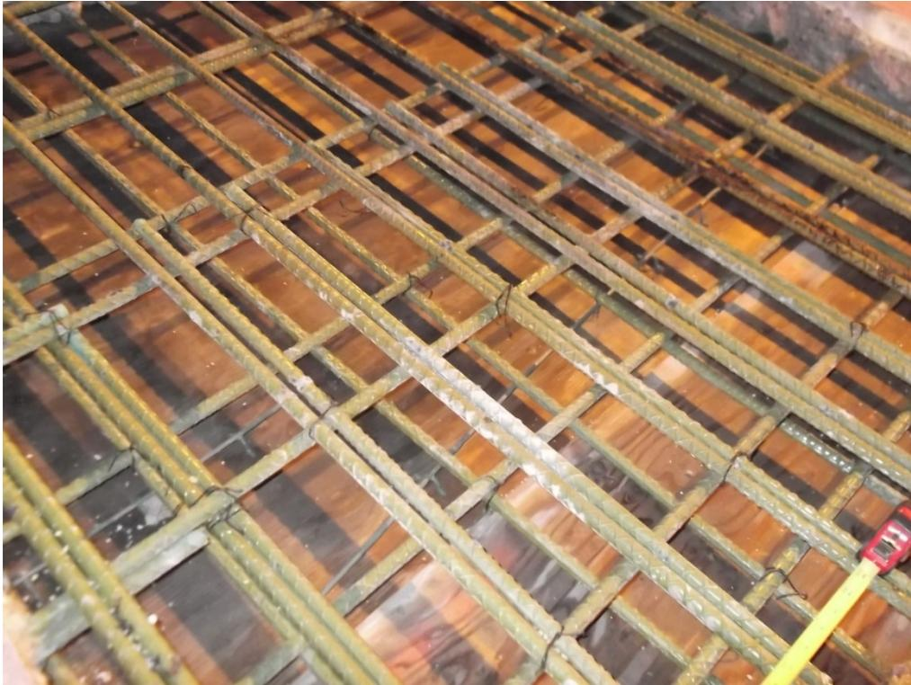
Fig. 4 – Layout of the reinforcement at the center of the patch.
